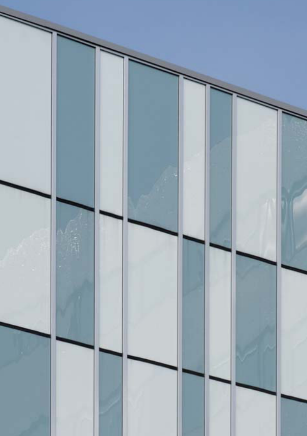
CHU Bordeaux, Pessac - Architectes : Gonfreville Lafourcade Roquette Photo : J.P. Lagarde
